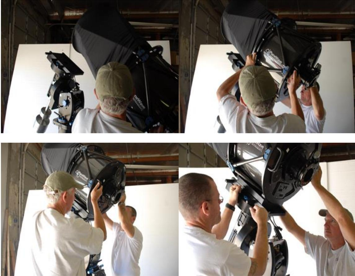
Figure 15 - Installation of a CDK17 onto an A200 mount using a PlaneWave 7.6" Saddle
