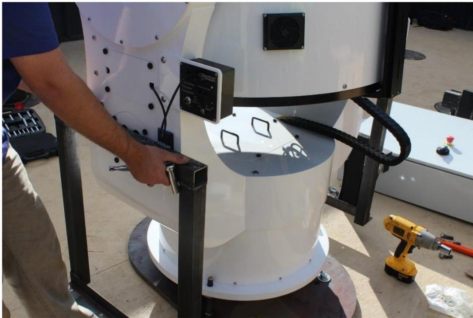
*Figure 20 Removing the shipping brackets*
