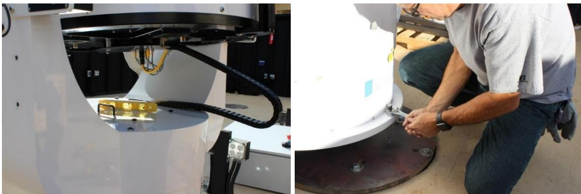
Figure 14 Leveling and securing the base
