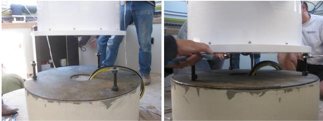
Figure 13 Lowering the base/fork assembly onto the threaded rods
