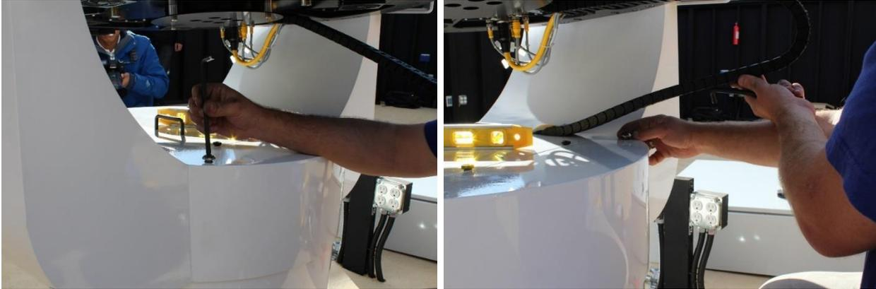
Figure 21 Removing the access hole covers
