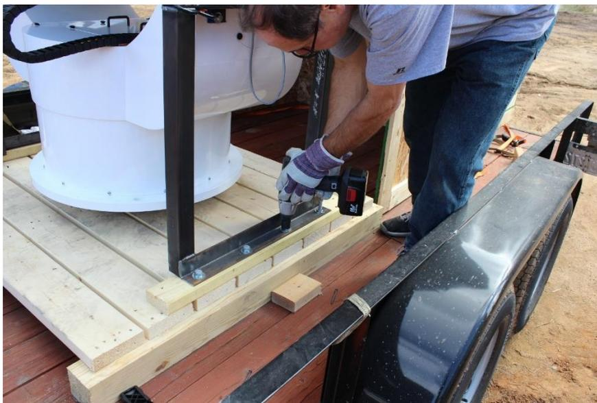
*Figure 4 Detaching the shipping brackets from the pallet*
