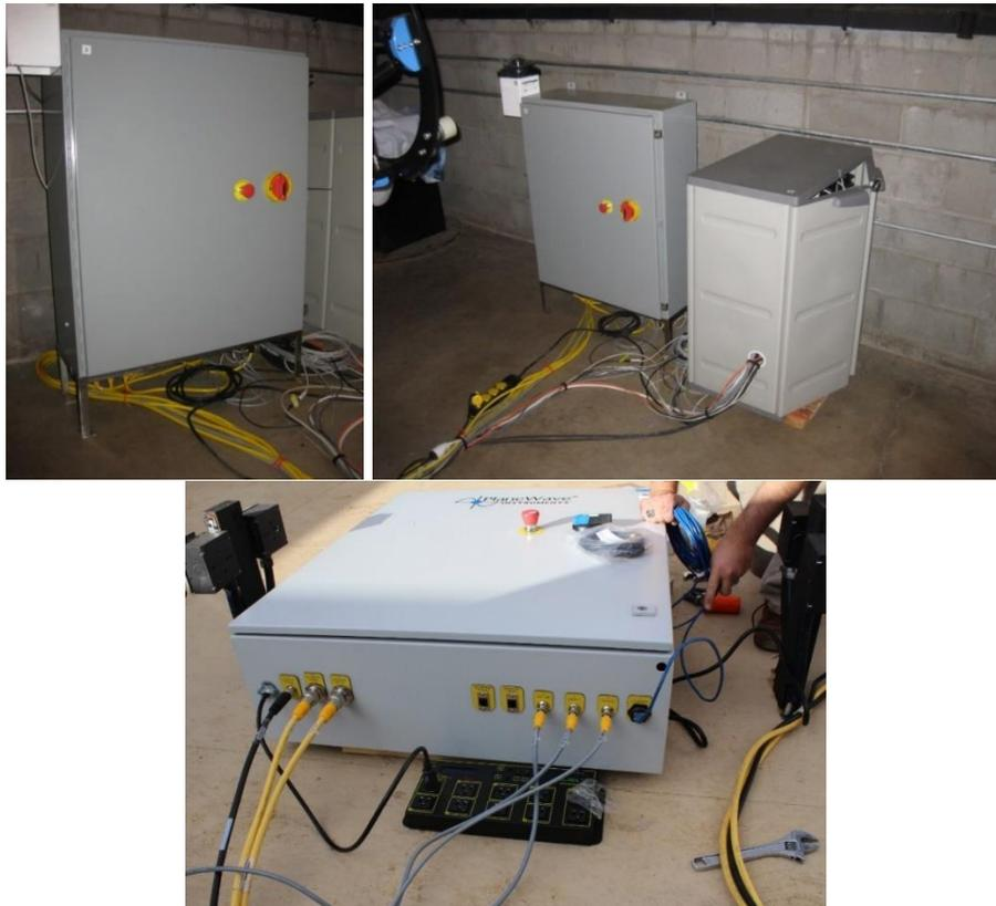
Figure 24 Control box mounting options
