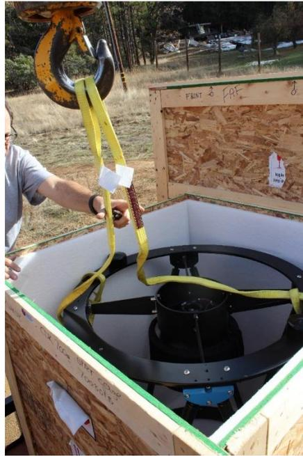
Figure 6 Upper cage ready to be lifted out of crate
