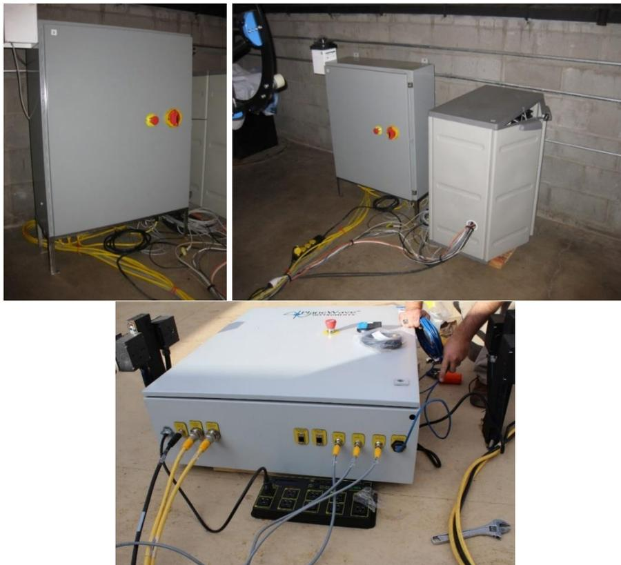
*Figure 24 Control box mounting options*
