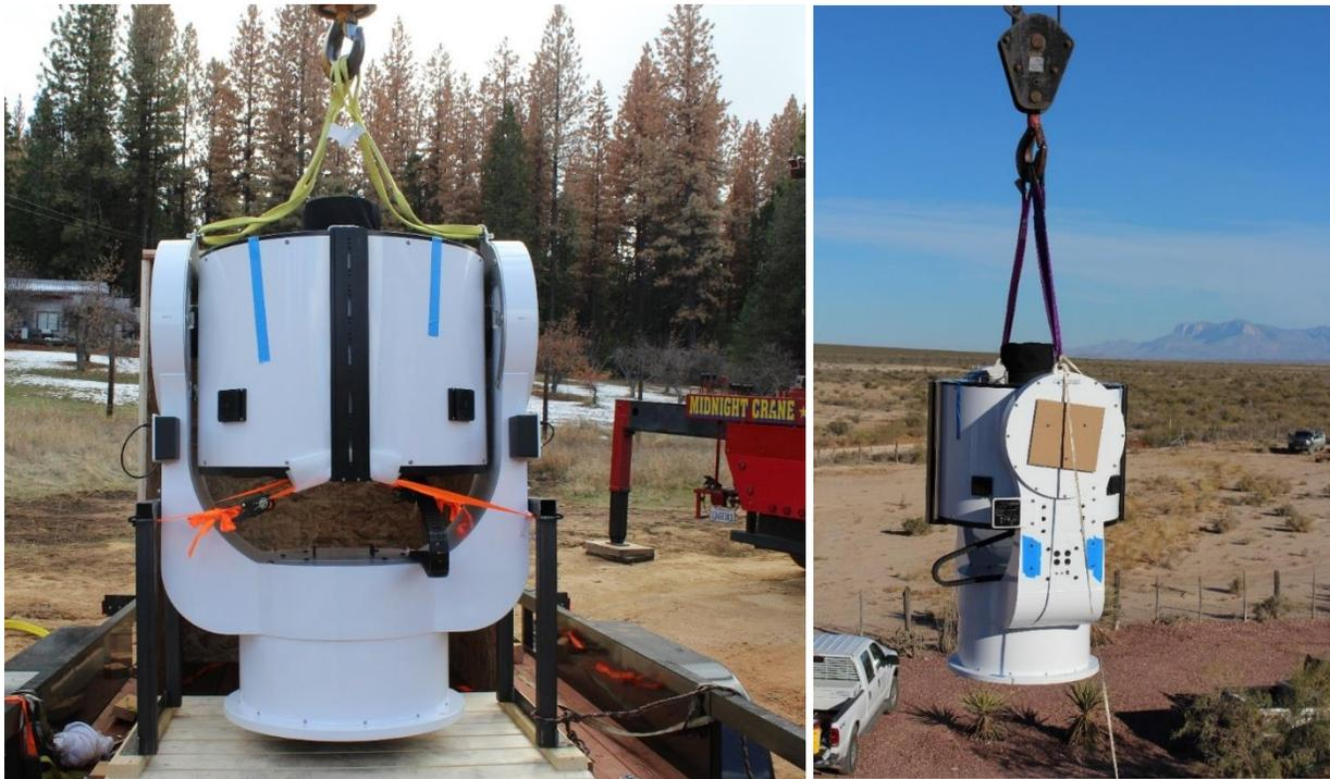
Figure 11 Lifting the fork into position
