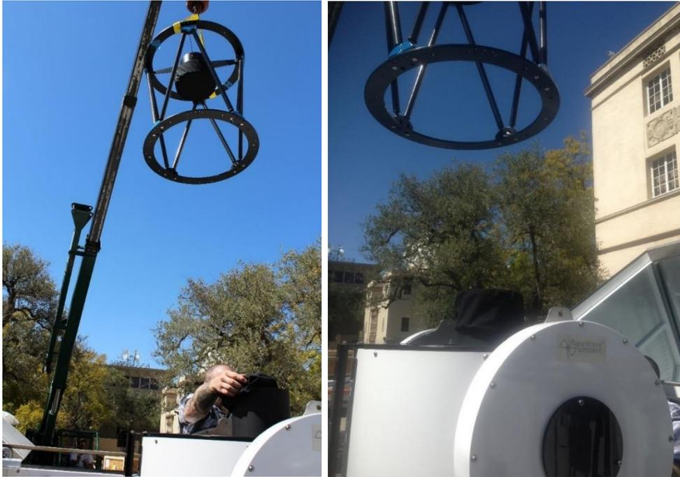
*Figure 15 Lifting the upper cage into place*
