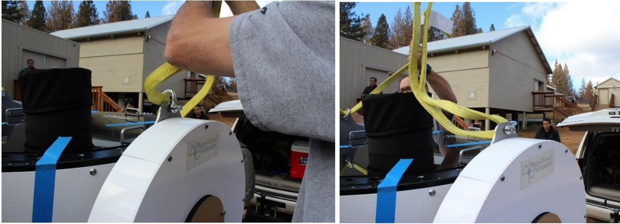
Figure 10 Rigging the fork for lifting
