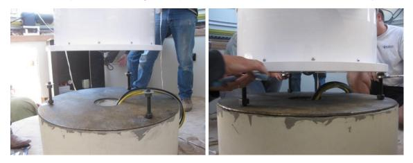
Figure 13 Lowering the base/fork assembly onto the threaded rods
