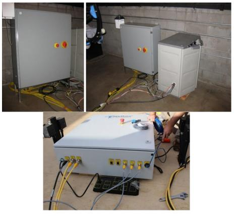
Figure 24 Control box mounting options
